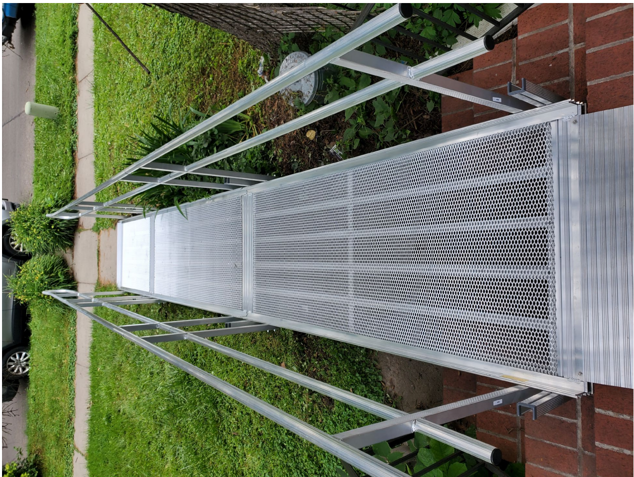
Installed aluminum ramp
