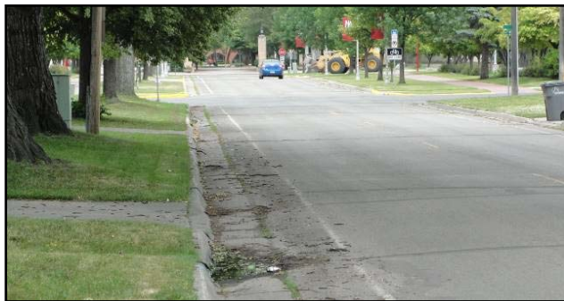
Debris in bike lane, Moorhead
