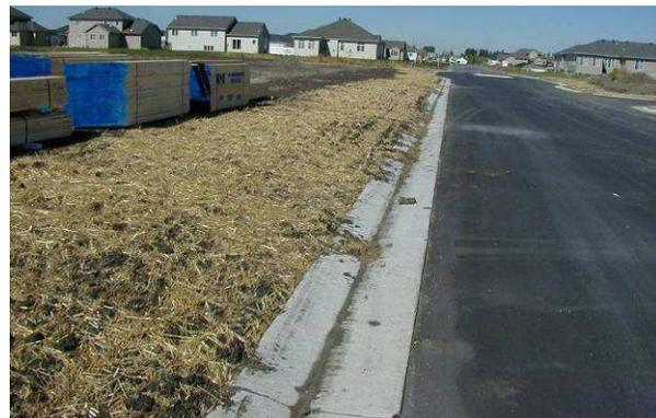
**Seed with Anchored Straw** (shown above) is also acceptable. The straw holds the soil in place until the seed germinates. It is critical that the straw be disk anchored, otherwise strong winds will blow the straw away from the area to be protected. Local landscaping firms offer this service.
