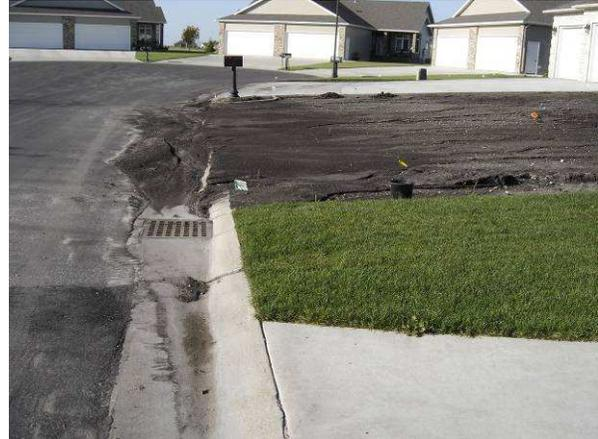
These two photos illustrate the need to stabilize the soil adjacent to the curb line when doing final lot grading and seeding. Each photo shows the **effectiveness of sod** on the boulevard of the lot in the foreground for eliminating erosion of sediments into the curb line. Note also the stormwater inlet in the right hand photo that has probably been polluted by the sediment from the lot in the background.
