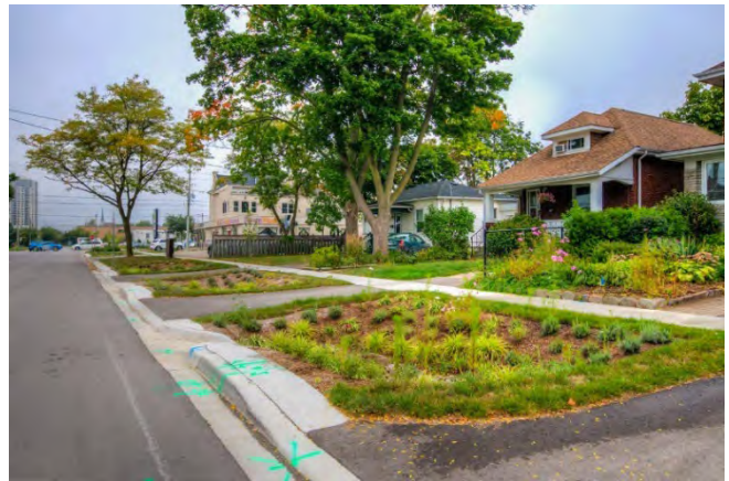
Example of Green Infrastructure (Credit: Stantec)
