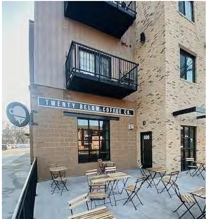
Photo of mixed-use building (Credit: Twenty Below Coffee Co.)
