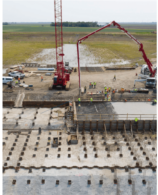
Diversion construction (Credit: Metro Flood Diversion Authority)
