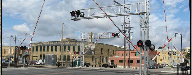
4-Quad Gate System 8th Street, Downtown Fargo
