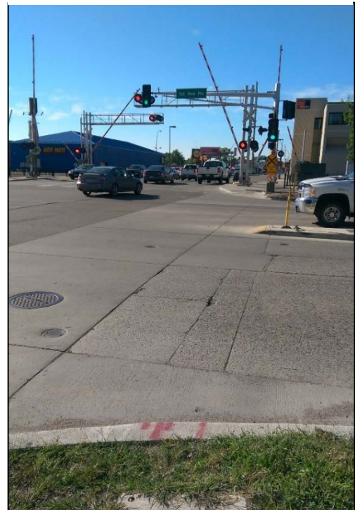
Figure 1 - Vehicles Clearing After a Train Event in Downtown Moorhead
