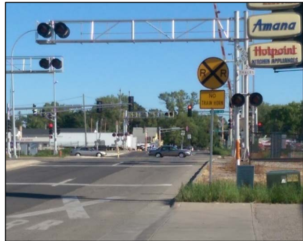
Figure 25 - Absence of Sidewalks along East Side of 14th Street
