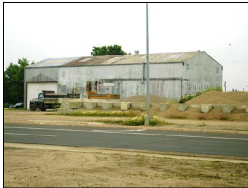
Unsightly building finishes, site, and complete lack of landscaping or boulevard trees.
