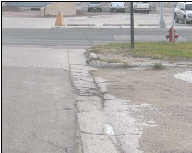
A curb and gutter in poor condition approaching 1 st Avenue N and along 1st Avenue N.
