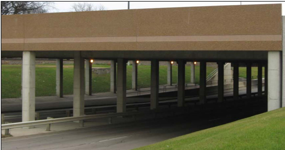
A sidewalk exists along the north side of 1 st Avenue N under the Moorhead Center Mall Parking Structure.
